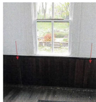
Figure D-15: Interior view of bell tower; evidence of original door location seen in area of replacement wainscot and cut in chair rail.
